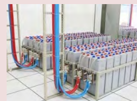
Basement of the building
