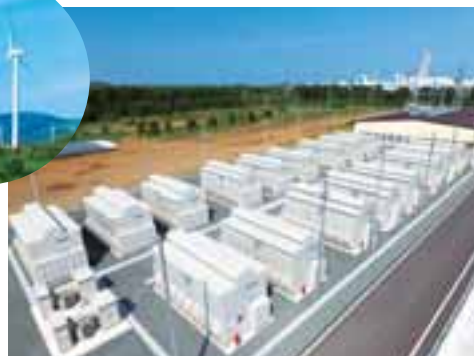
NAS® battery system for large-capacity power storage
