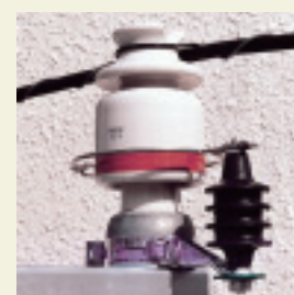
Distribution insulator and Current Limiting Arcing Horn
