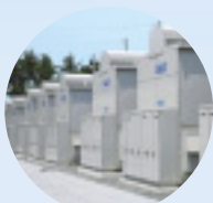
NAS batteries for power storage
