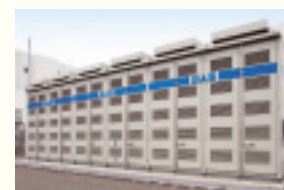
NAS batteries at the Nagoya Site
