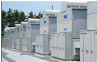
NAS battery systems for electric energy storage
