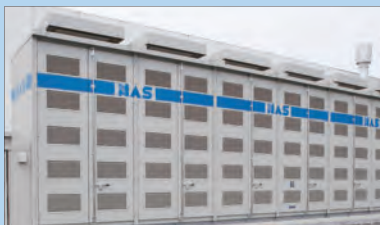
NAS ® battery systems for electric energy storage
