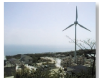
Starting in March 2001 in Hachijojima, Tokyo Electric Power Company (TEPCO) has been entrusted by the New Energy and Industrial Technology Development Organization (NEDO) to conduct testing of NAS batteries in conjunction with wind power generation facilities.
