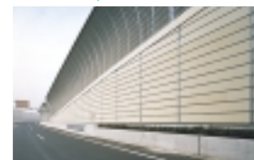
Sound-absorbing boards made of ceramic fragments
