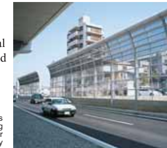
HISHUT in use as a sound-absorbing material for an expressway
