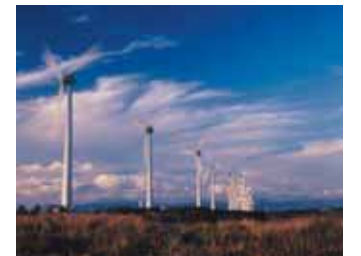
The Noshiro Wind Power Station
