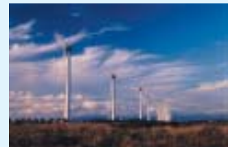
The Noshiro Wind Power Station
