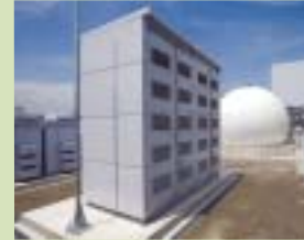
NAS® batteries electrical storage system
