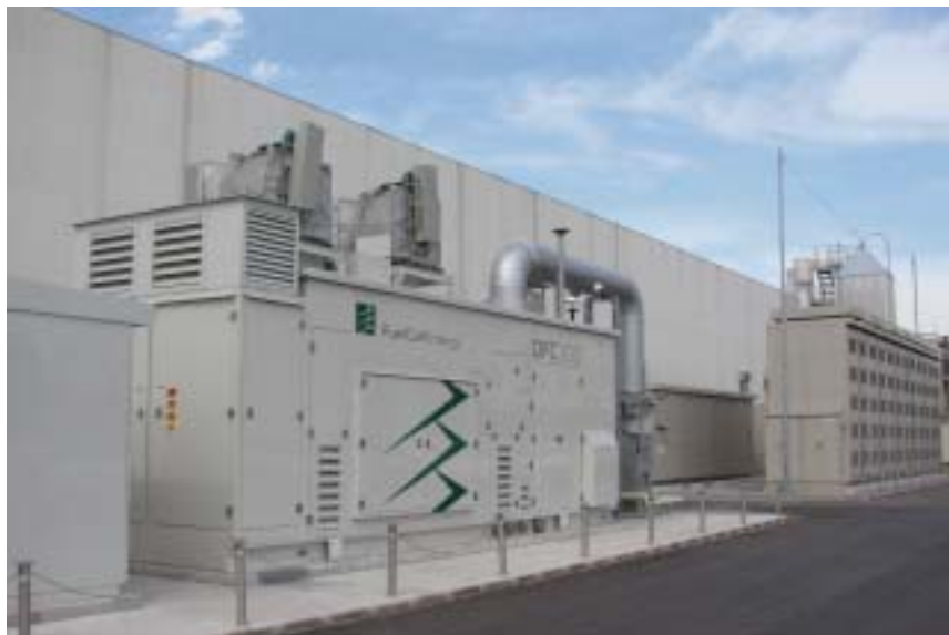
System combining fuel cells (front) and NAS ® batteries (rear).
