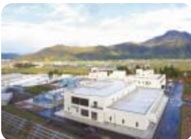
Aerial view of the water purification facility
