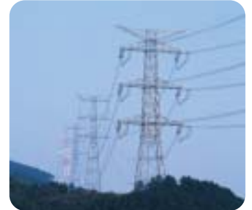
Insulators for power lines
