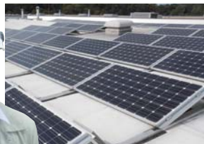
255 solar panels installed on the roof of the plant
