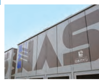
There are already approximately 200 working examples of the NAS battery in Japan and overseas.
