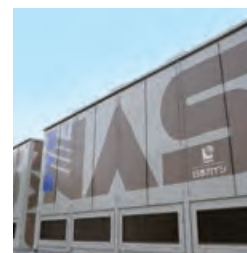
NAS battery which is the first megawatt-class electric energy storage system being utilized in the world
