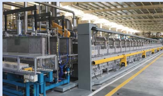
Roller hearth kilns
