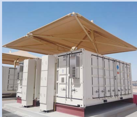
NAS batteries installed in Dubai
