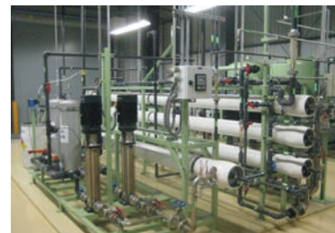
Filtration device using reverse osmosis membranes
