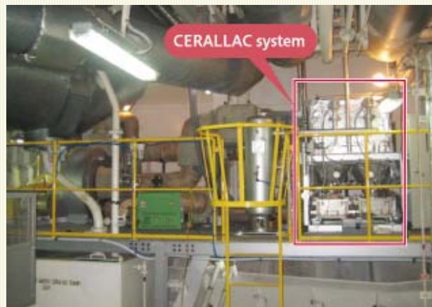
Confirming high PM removal performance during a demonstration test on a marine vessel
