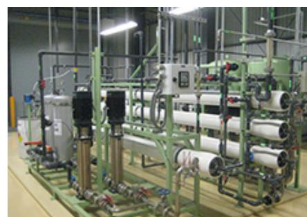
Filtration device using reverse osmosis membranes
