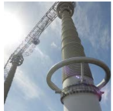
The world's largest 11 meters hollow insulator for substation systems. Our advanced design and manufacturing technologies have been applied to achieve long-term performance which resist up to 1,000-kV-power transmission systems and massive earthquakes.
